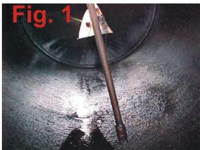
In Figure 1, there is shown a 1,000 gallon underground fuel storage tank containing jet fuel residue and flammable vapors. Before this tank could be dismantled with cutting torches, the remaining fuel needed to be neutralized and the tank thoroughly cleaned to remove any flammable
